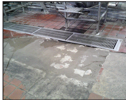
Facility D—Kitchen Floor Tiles
