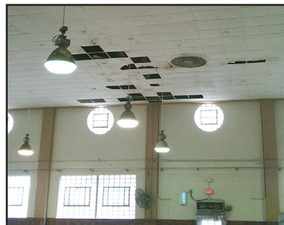
Facility D—Dining Hall Ceiling
