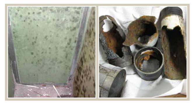
Sources: Photographs by Hygiene Technologies International, Inc., and the California Department of General Services' building manager. Note: Visible mold (left) and corroded drainage pipes (right).
